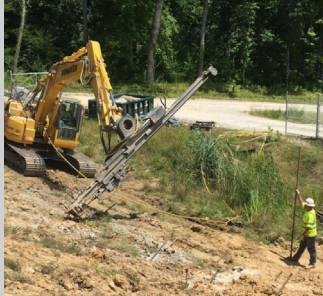
NAVFAC Crane Earthen Slide Repair
