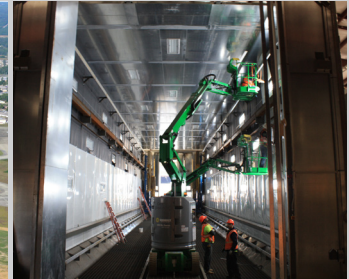
UPRR DeSoto Blast Building
