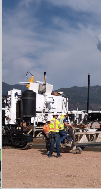
Alpha Ramp Replacement Fort Carson
