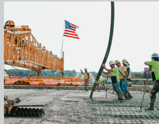
MoDOT I-270 North DB
