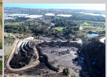
Santa Barbara Debris Removal
