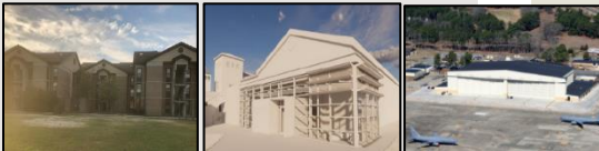
FT BRAGG BARRACKS RENO. | FT BRAGG INNOVATION OUTPOST | SEYMOUR J. AFB KC46A HANGAR
