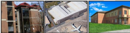
FT STEWART VOLAR BARRACKS | ROBINS AFB PAINT/DE-PAINT HANGAR | ROBINS AFB ABMS OPS FAC.
